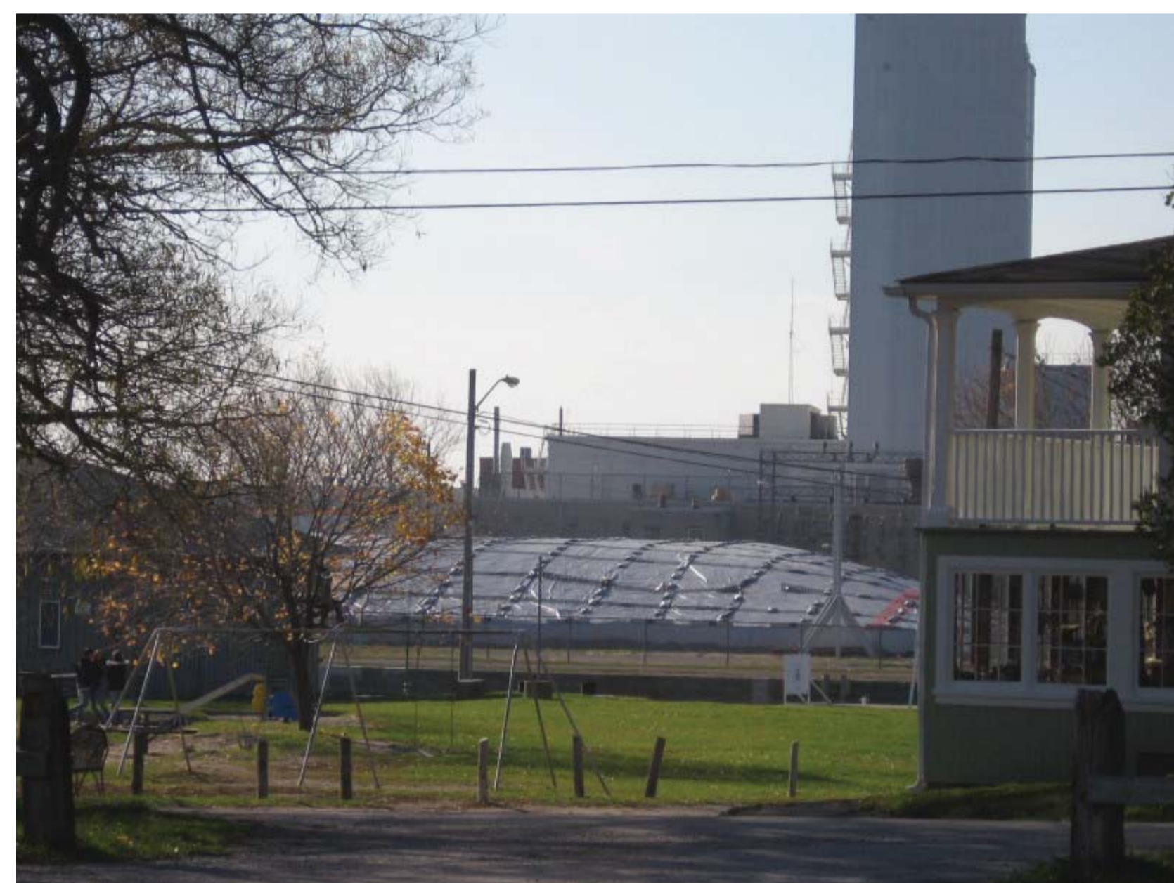
A street, private home, and children's playground in the immediate vicinity of the Cameco facility; a tarp covers uranium tailings
